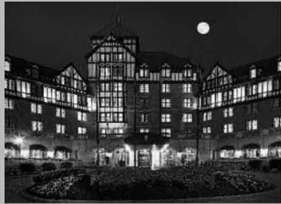
The Hotel Roanoke at Night
