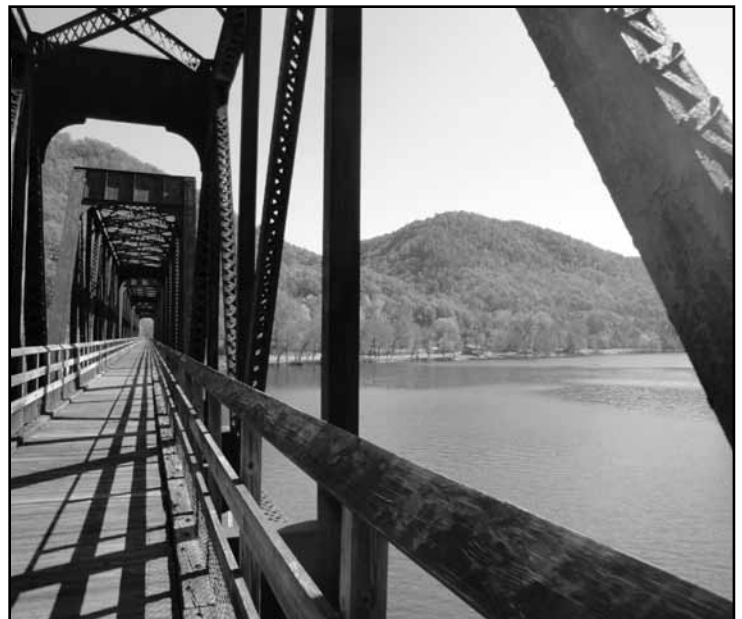
951 Foot Bridge in Hiwassee
